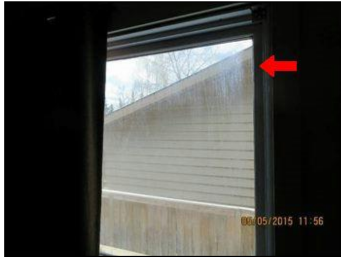
18. Excess condensation
