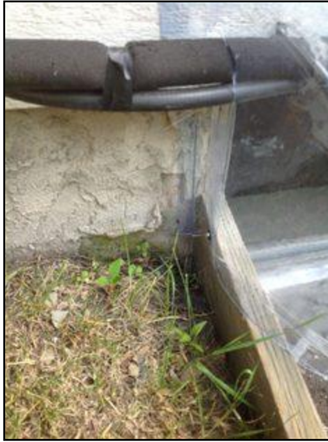
7. Parging damaged or missing
