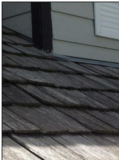
4. Damage, loose, open seams, patched
