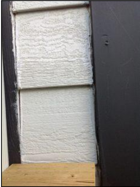
5. Missing paint or caulking
