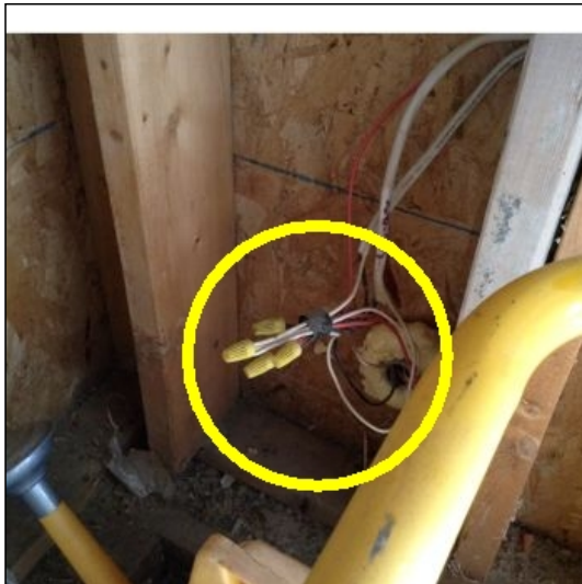
All wires should be in sealed junction boxes
