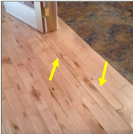
Separation noted on dining area - No humidifier will not help
