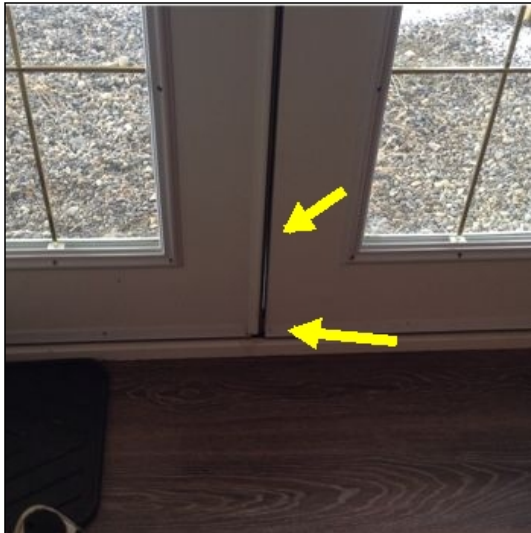
Replace weatherstripping to reduce heat loss at exit doors
