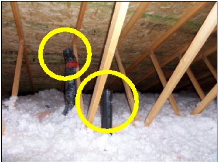
Should be externally vented
