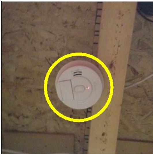
All tested and worked as required - due to age replace all and add carbon monoxide detectors
