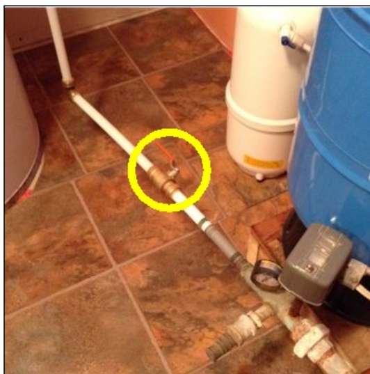
Water shut off to feed
