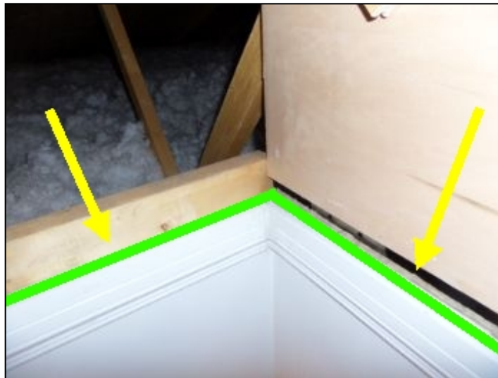
Add weatherstripping at attic hatch
