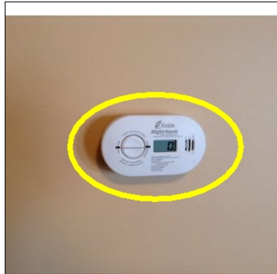
Carbon monoxide detector in place
