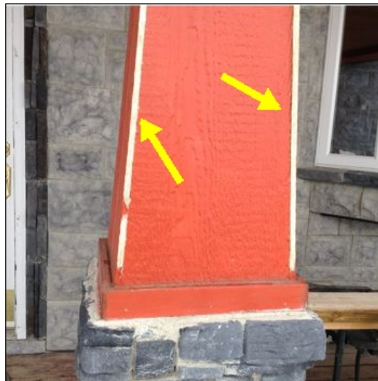
Scrape and repaint as required
