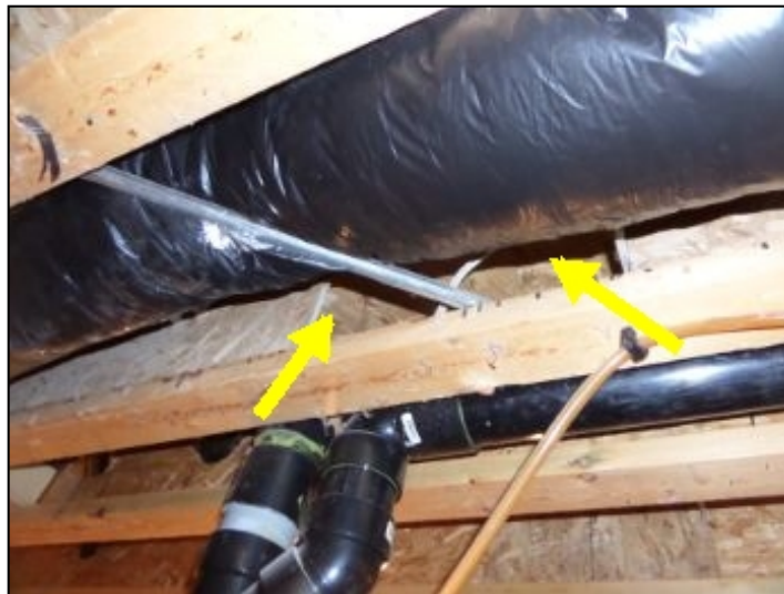
Over cutting weakens the floor joists
