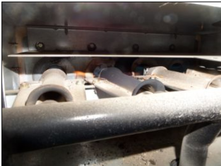
Flame not even - possibly problem - hvac engineer to inspect
