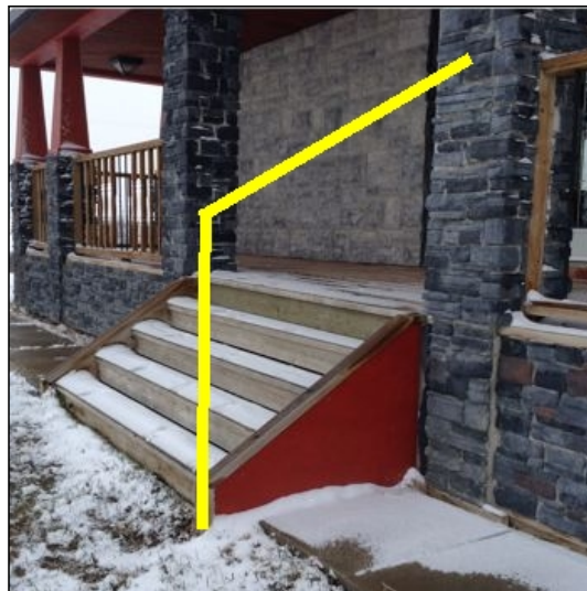
Add handrail at steps as required
