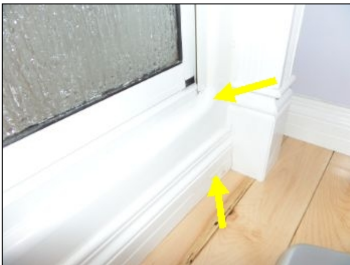
Slight leaking at shower in en suite 2
