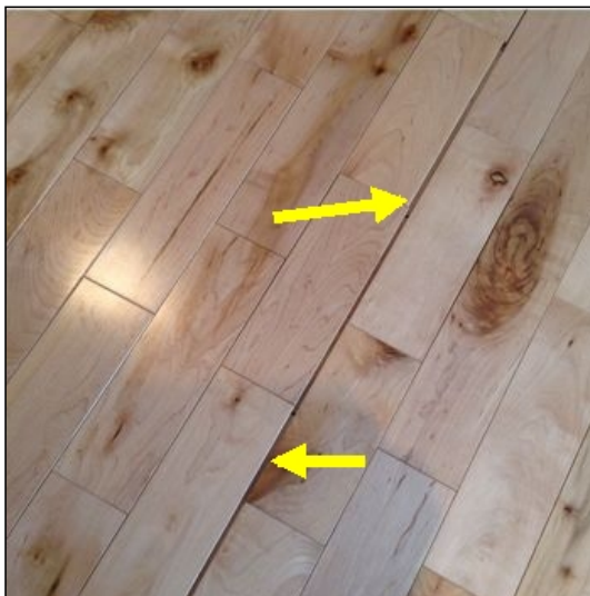
Slight floor separation noted in bedroom 2
