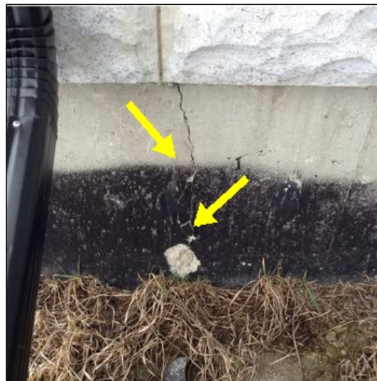
Common shrinkage cracks noted
