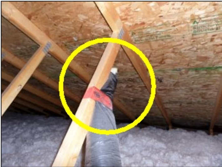
In correct venting can cause moisture and mold issues
