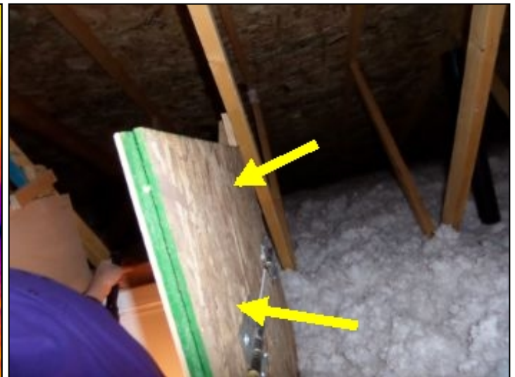
Add insulation to attic hatch
