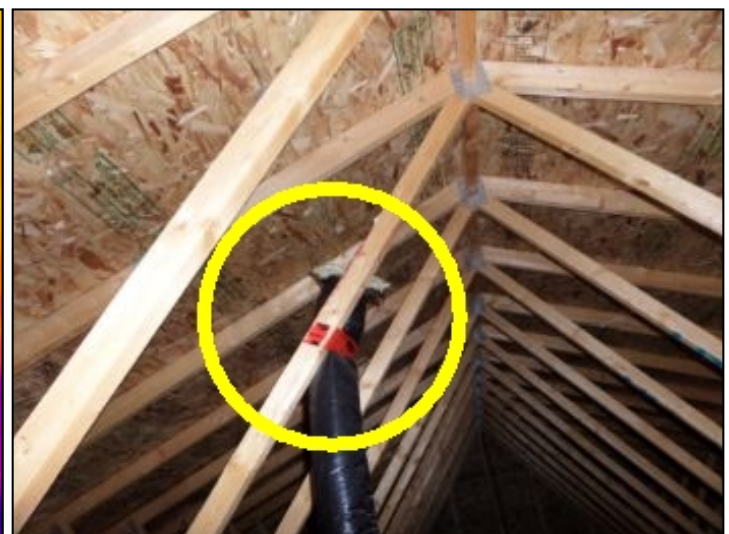
exhaust fan is vented into attic area - must vent externally
