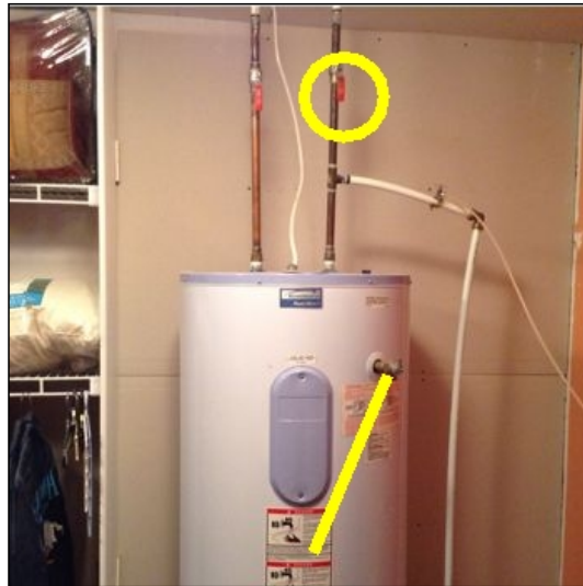
Water shut off to tank - add pressure relief valve
