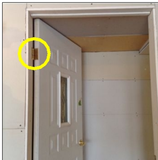
Door into garage should self close for safety
