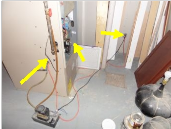
No kill switch for furnace and powered with extension cord
